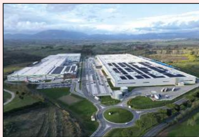
A Segro warehousing hub in Italy
