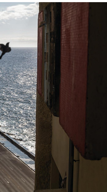
Seen between the weathered facades of the Girón apartments, a lone car moves along the Malecón, once a vital artery
